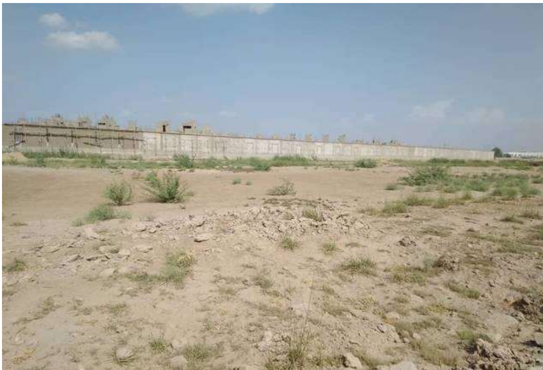
Figure 2: Current Status of Proposed Project Site – Pic 2
