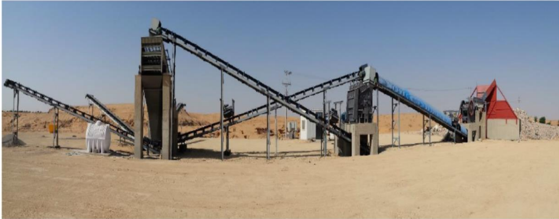
Figure 3.12: C&D recycling plant
