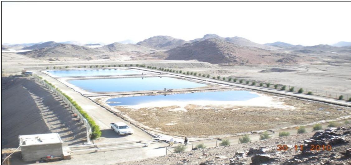
Figure 3.19: View of Three Stage Leachate Treatment System
