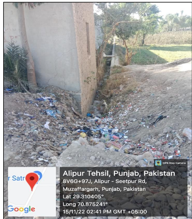
Solid waste clogging sewage channels in Ghouspur
