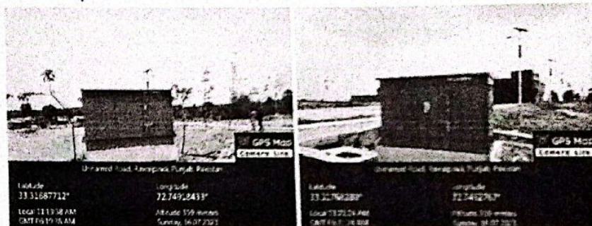
FIGURE 3.3: LOCATION OF TRANSFORMERS AT THE PROJECT SITE.
