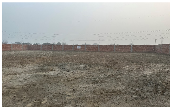
A view of the Boundary wall of proposed factory of MSI Engineering Services
