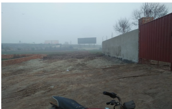
An outer view of the proposed factory boundary wall of MSI Engineering Services at Mehmood Booti
