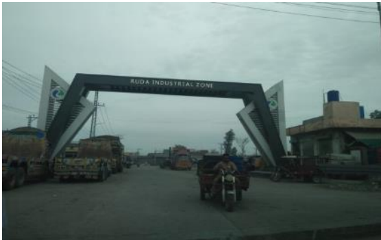
A view of Main Gate of Existing Industrial Zone of RUDA at Mehmood Booti.
