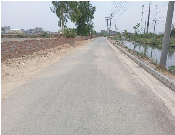
Exhibit 5.3: View of access road to the project site
