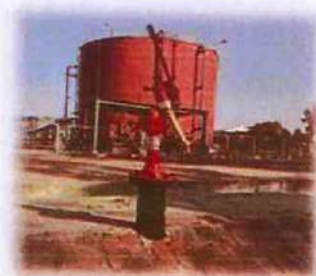
Single barrel fixed water monitor
