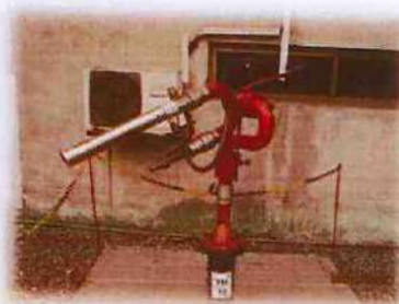
Double barrel fixed foam monitor
