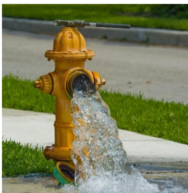
Figure 11-10 Fire Hydrant
