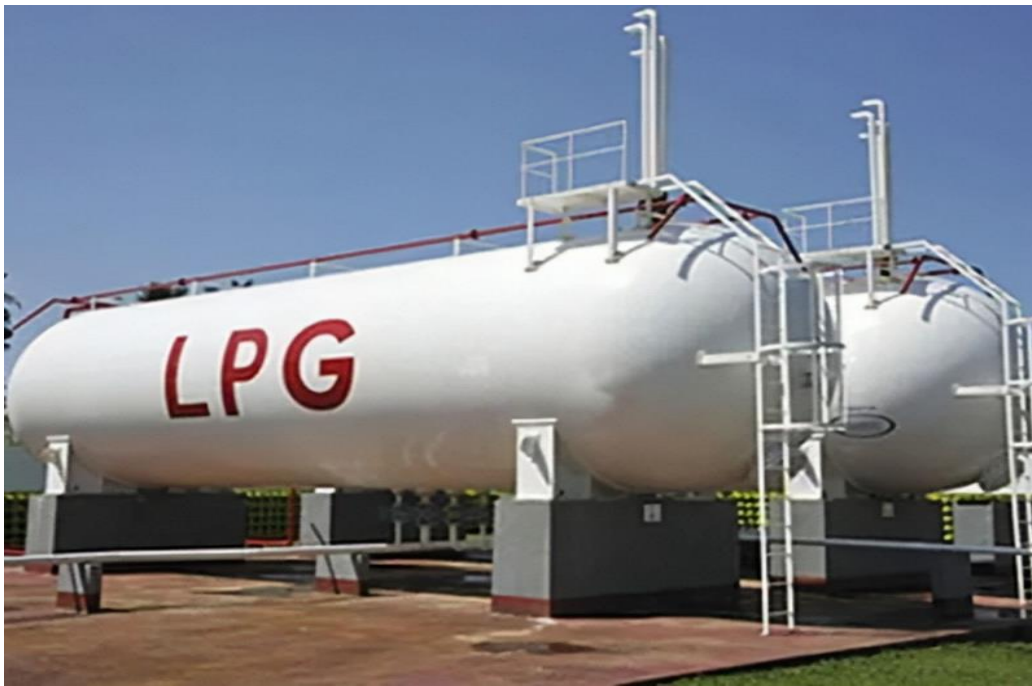
Figure 5-3 Storage tank Design
