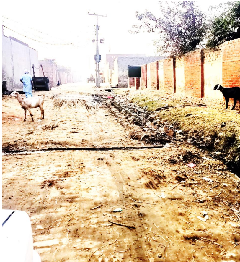
Figure 3.10: Sanitation & Drainage in the project area
