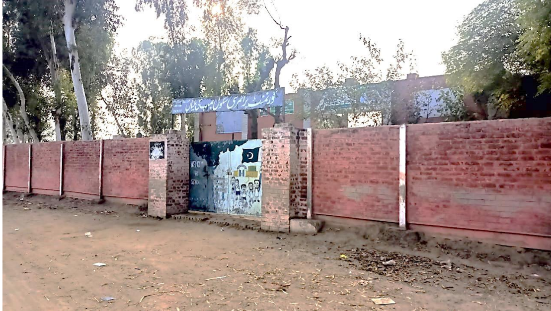
Figure 3.16: A primary school at Bhamb Ki Mallian Village
