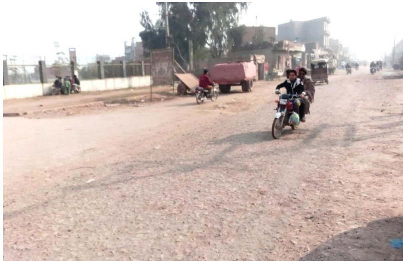
Figure 3.14: Condition of roads inside Sheikhupura City
