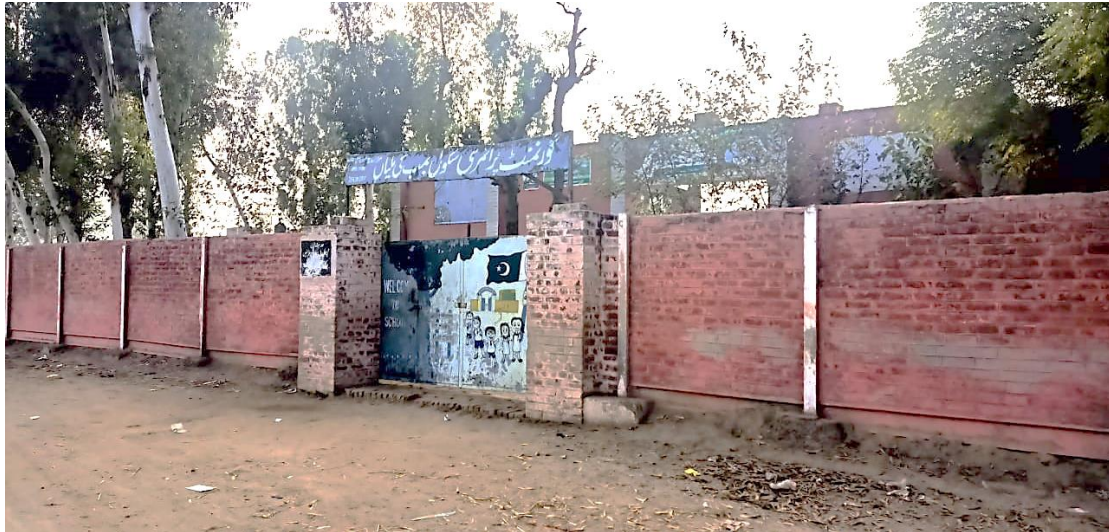
Figure 3.17: A primary school at Bhamb Ki Mallian Village
