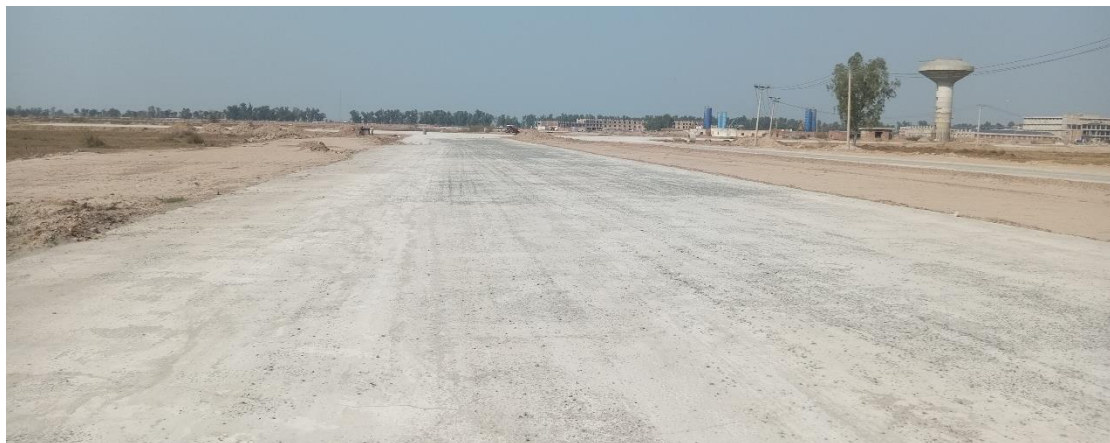
Figure 3.15: RCC roads under development at QABP, Sheikhupura
