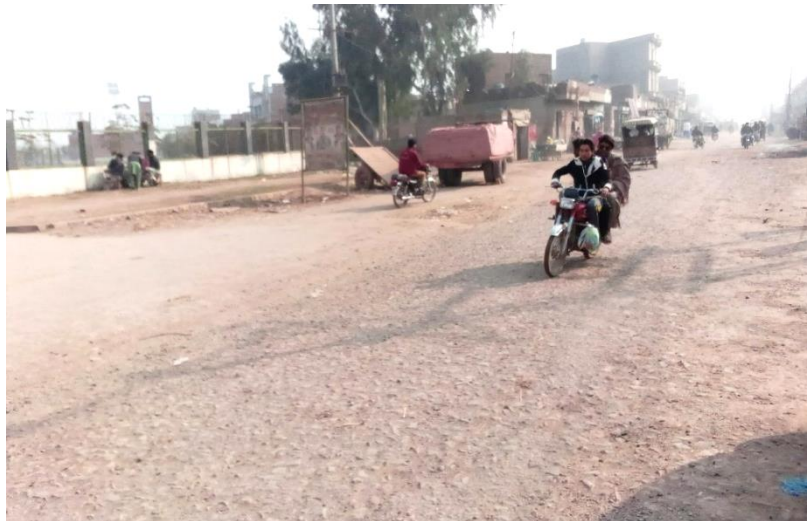
Figure 3.14: Condition of roads inside Sheikhupura City
