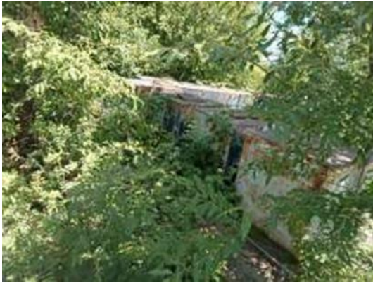
Photo 82: Water Storage Tanks
