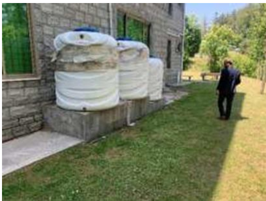
Photo 78: Water Storage Tanks
