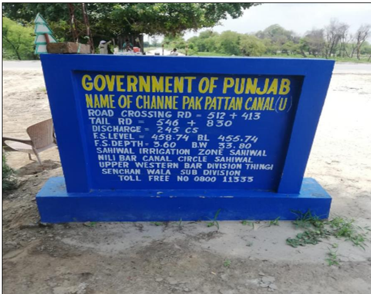
Figure 6-13, Discharge of Pakpattan Canal in Vehari Area
