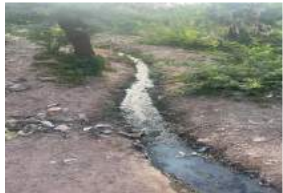
Drain Channel Falling in the River
