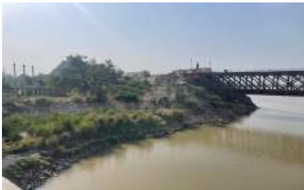
Bridge Over Chenab River and Transmission Lines
