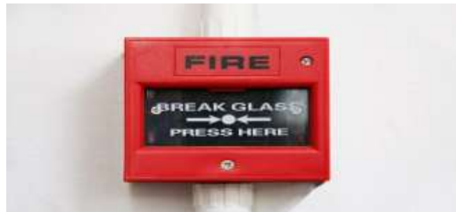
Figure 10-11 Fire Alarm
