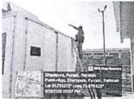
Figure 7: Stack Emission Monitoring of Generator 2
