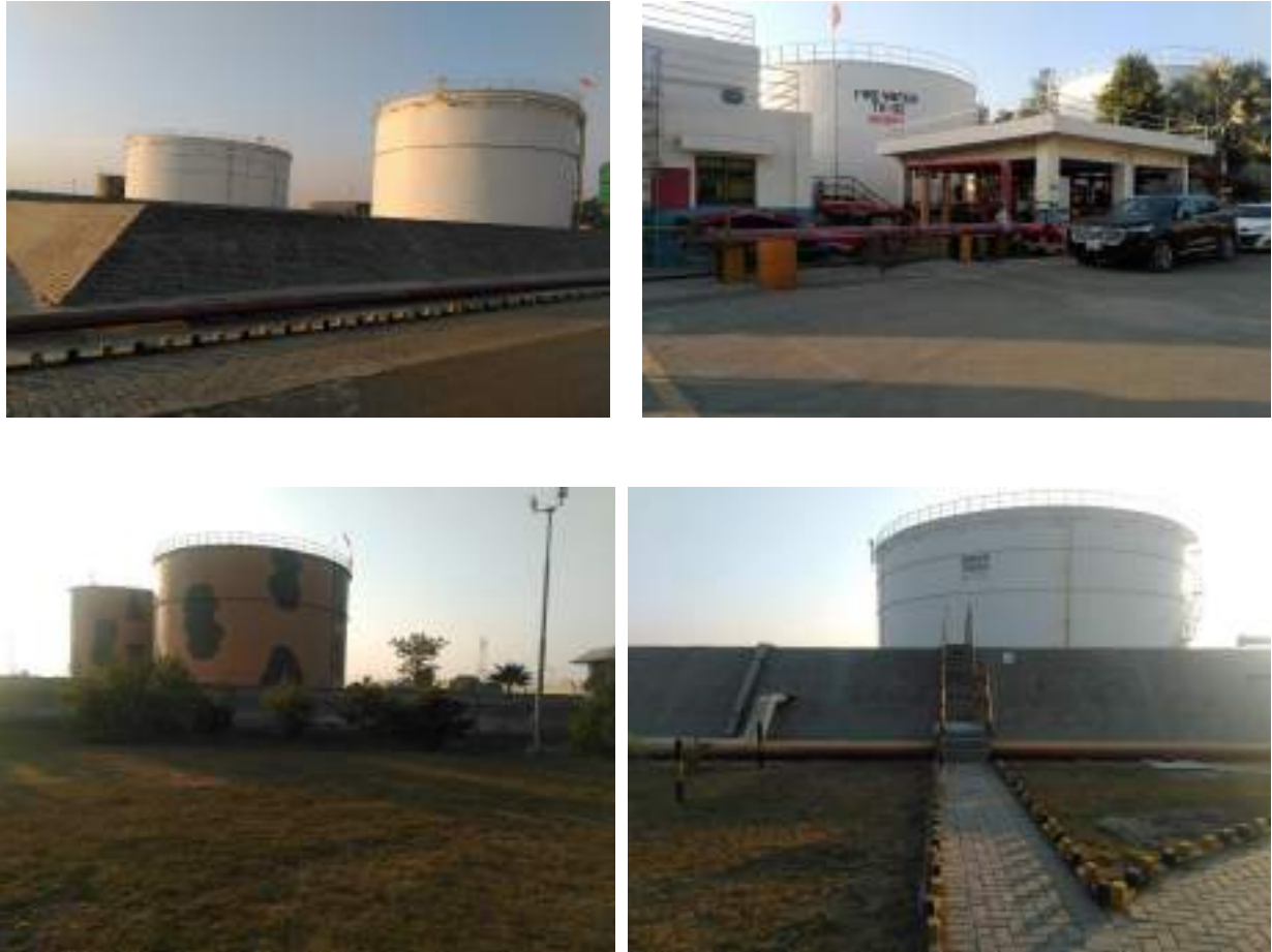
Figure 4-6 Tanks at the Project Site
