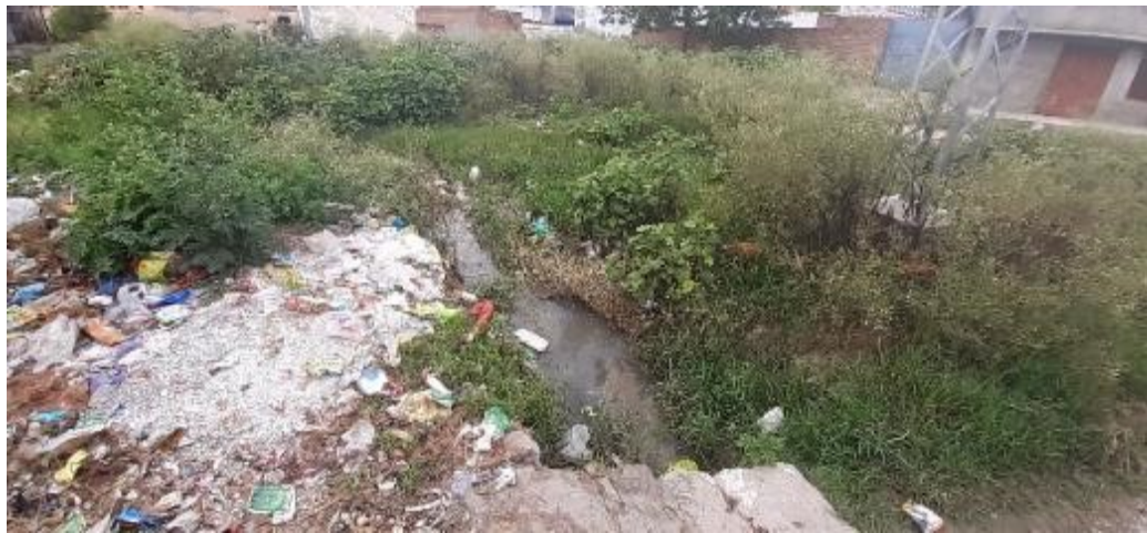
Figure 4.12: Open channel for Sewage water in a village in Adhi ML
