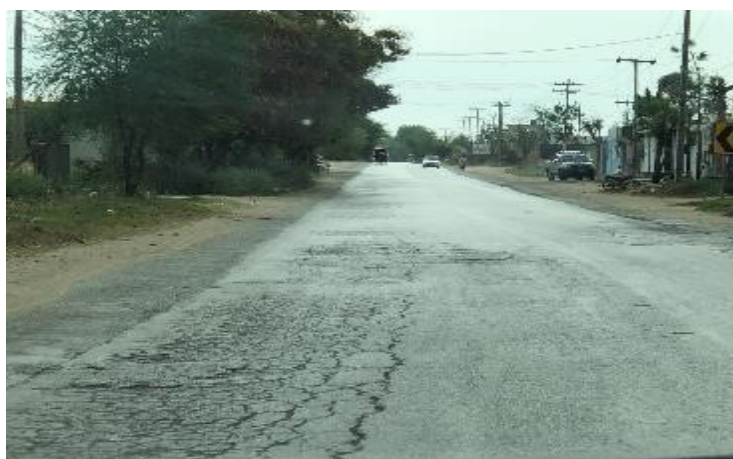
Main Doltala - Rawalpindi Road
