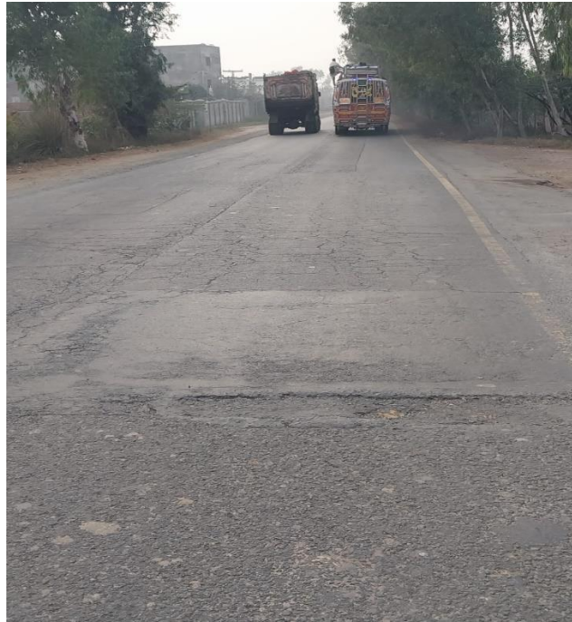
P.P 3.2: view of access road, Muridka- SKP road
