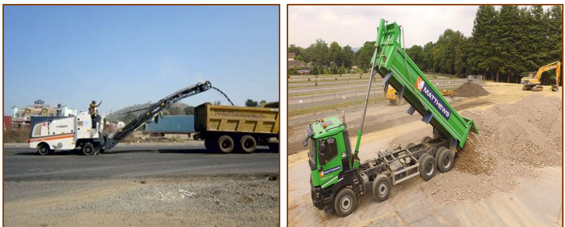
FIGURE – 11.4 : MACHINERY USED FOR DISPOSAL OF MUCK
