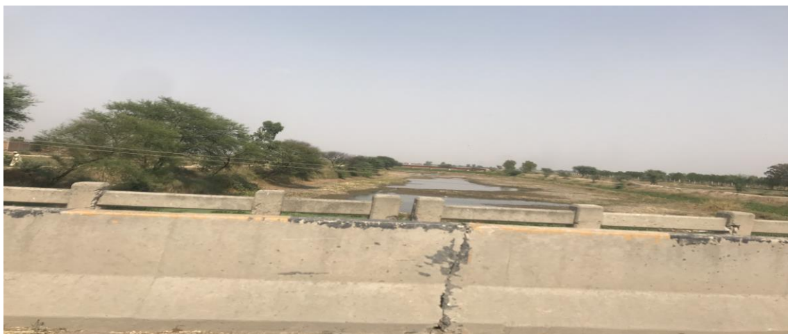
Figure 6-7 Ninki Degh Canal Sheikhupura
