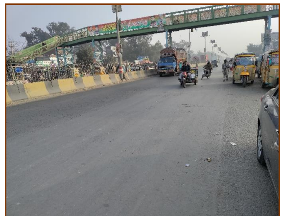
PEDESTRIAN OVERHEAD CROSSING NEAR SADHOKE (KM. 1299+000)
