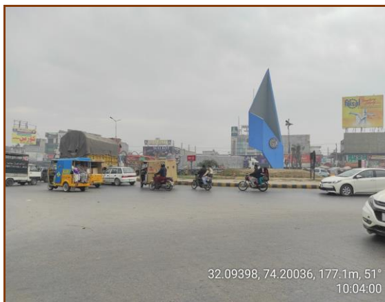
CHAND-DA-QILA ROUNDABOUT (KM. 1320+300)
