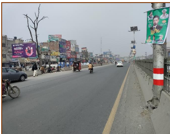
MURIDKE BUILT-UP AREA (KM. 1286+000)
