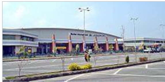
Figure 10 Multan International Airport
