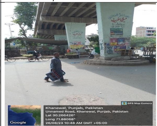
Start point of Islam building sewerage scheme
