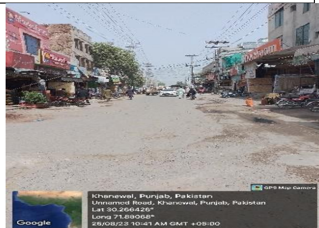
View of road
