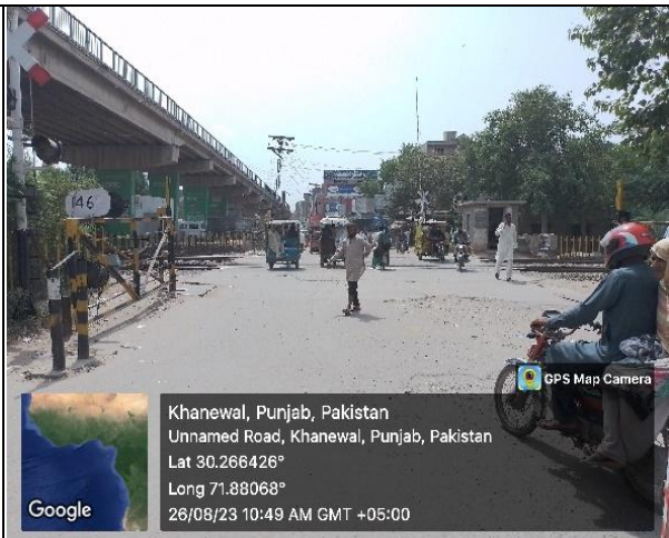
Sewerage crossing railways line
