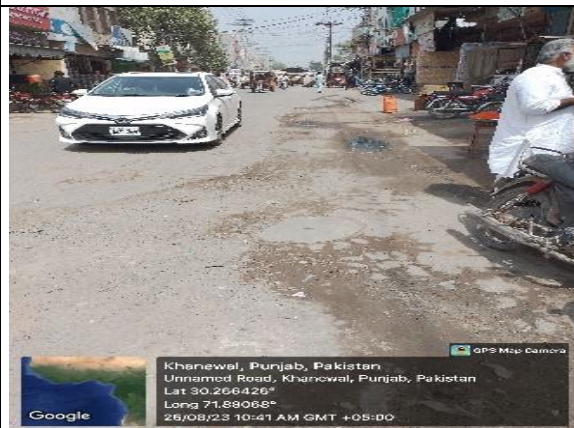
View of road
