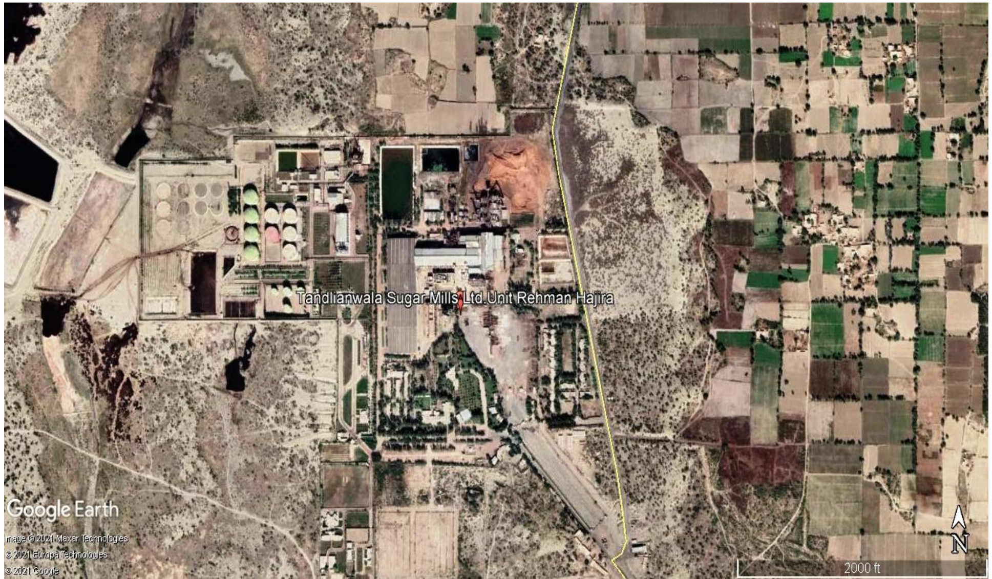
Figure 5-1 Google View of Tandlianwala Sugar Mill & Distillery Unit Rehman Hajira
