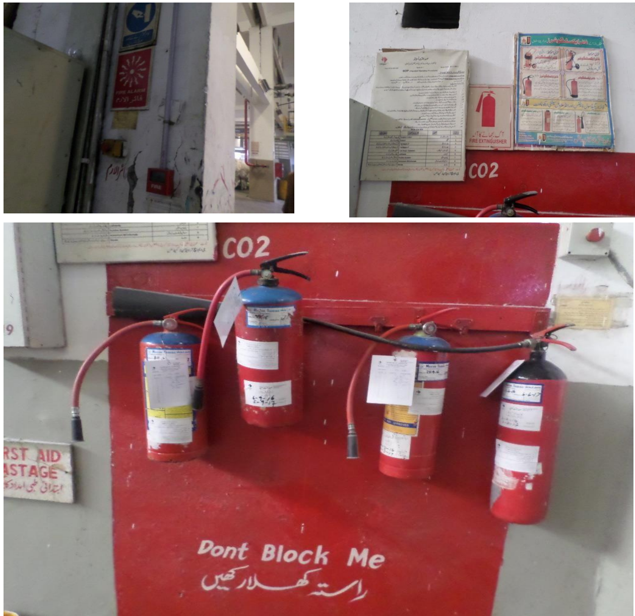
Figure 11: Pictorial view of fire alarm system at existing unit
