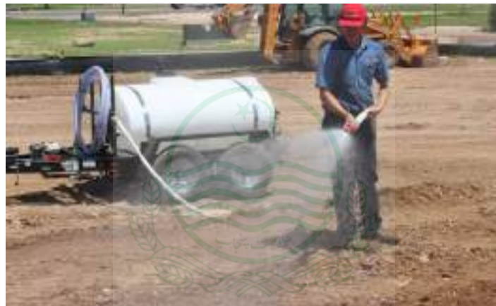
Figure 7-3 Water Sprinkling
