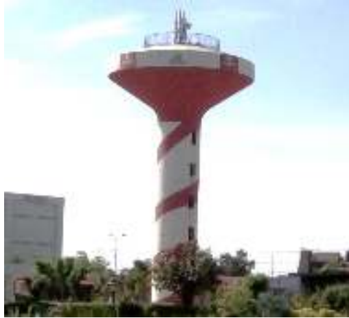
Figure 3.6: One of the Overhead Water Tanks installed throughout SIE
