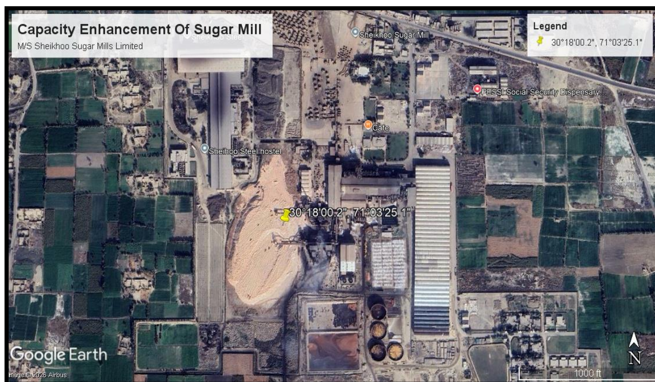
Figure 1. Aerial view of the project site
