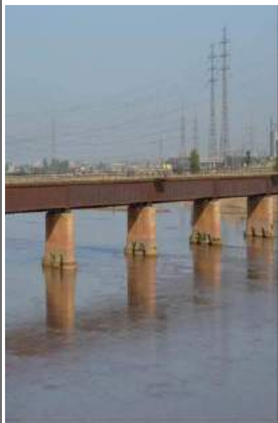
Shahdara Railway Bridge
