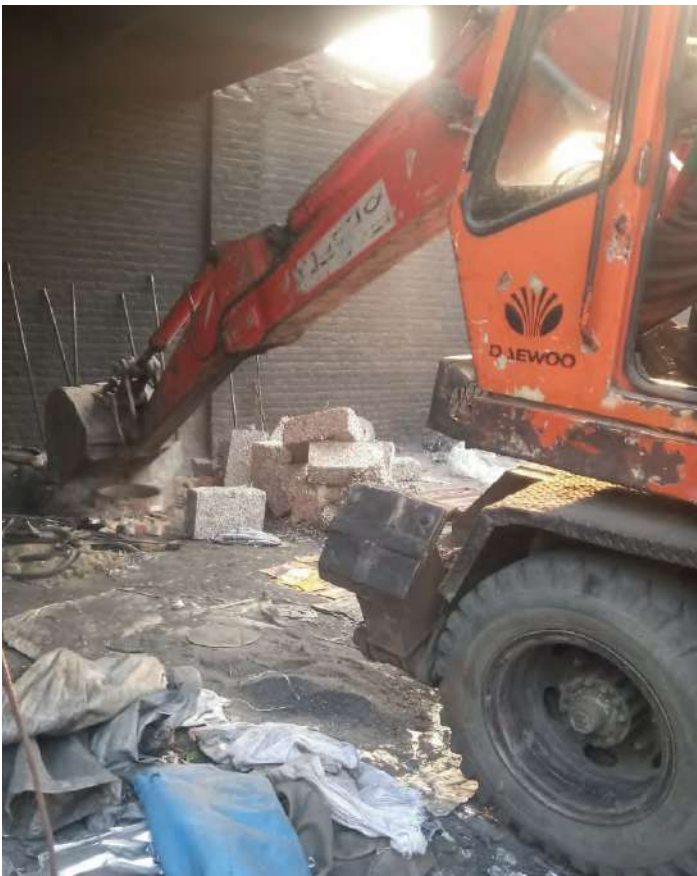
Demolition of Industry
