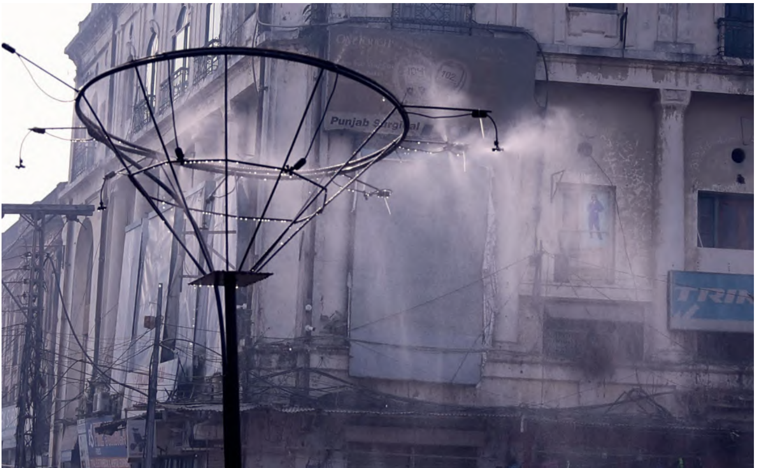
Mist Sprinkler System
