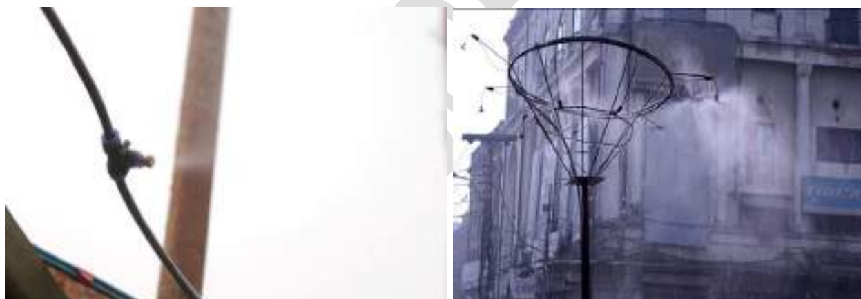
Figure 5.26: Mist Sprinklers installation at under construction sites
