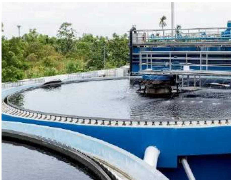
Figure 6.6: Waste Water Treatment Plant
